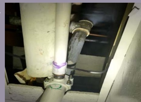
Sanitary Sewer Line Above Suspended Ceiling
